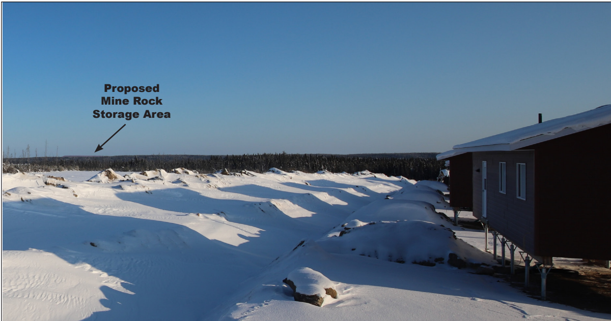
Photo 15A-2: View of future Project infrastructure at Gordon site looking north from Black Sturgeon Reserve vantage point
